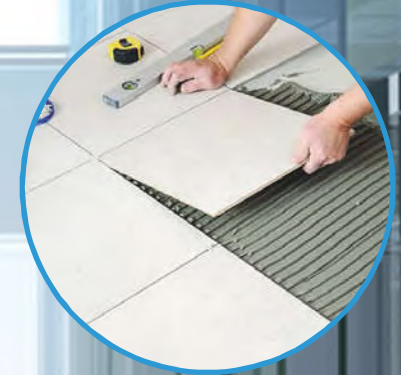
Tile/ Marble & Epoxy Coating
